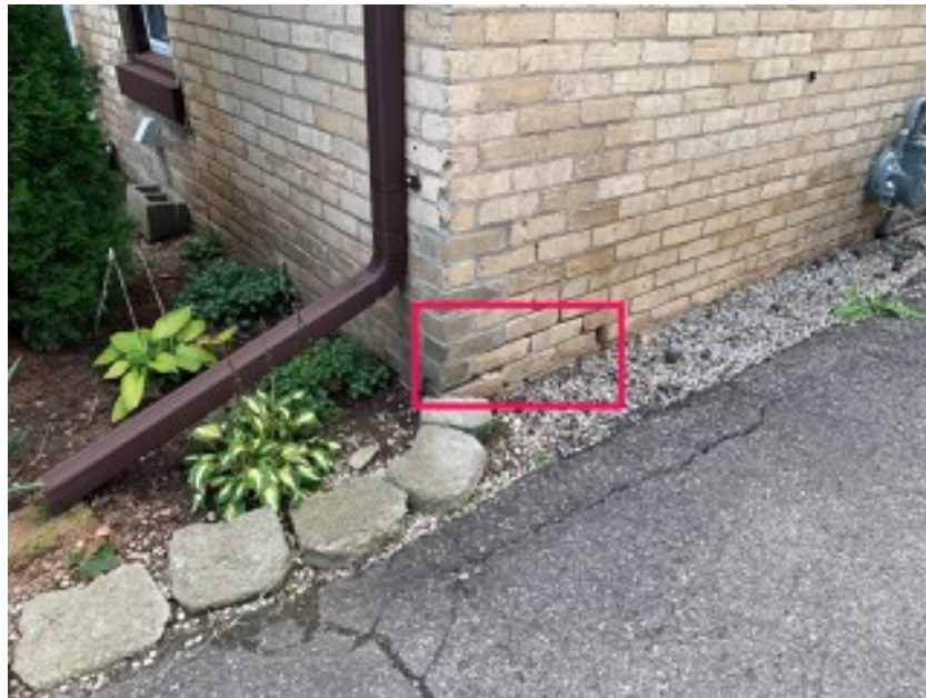
Figure 6: Repointing work proposed for side (east) facade. Source: Stonebridge Masonry.
