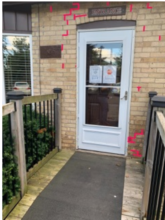
Figure 8: Repointing work proposed for area around rear entrance. Source: Stonebridge Masonry.
