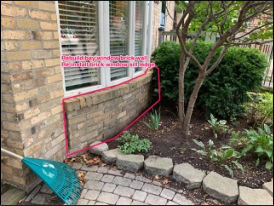
Figure 4: Rear bay window knee-wall to be rebuilt. Source: Stonebridge Masonry.
