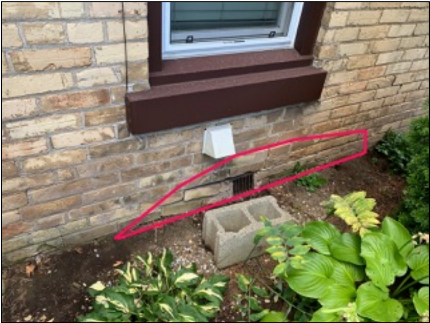
Figure 4: Rear bay window knee-wall to be rebuilt. Source: Stonebridge Masonry.
