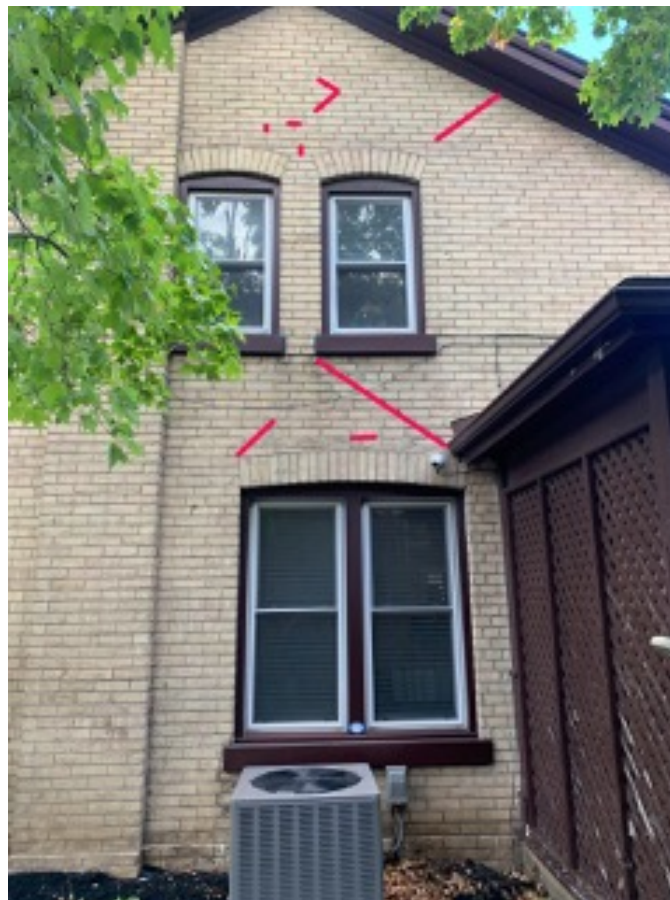
Figure 6: Repointing work proposed for side (east) facade. Source: Stonebridge Masonry.
