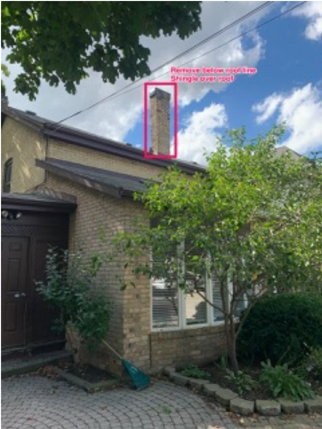
Figure 11: Chimney at rear of building proposed to be removed. Source: Stonebridge Masonry.
