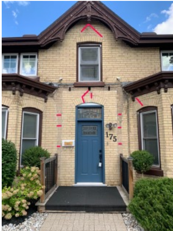
Figure 10: Repointing work to occur around front entrance. Source: Stonebridge Masonry.
