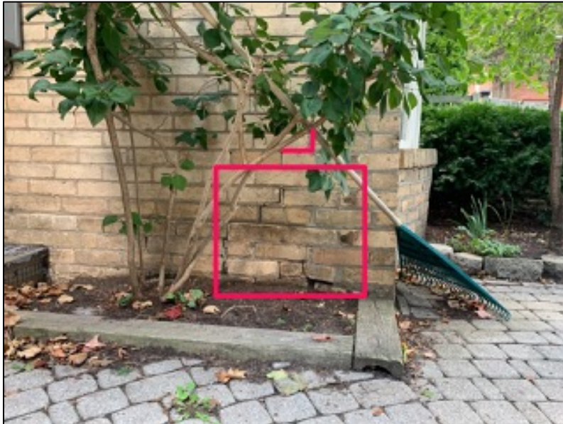
Figure 2: Repointing work at front (north-west) corner of building. Source: Stonebridge Masonry.
