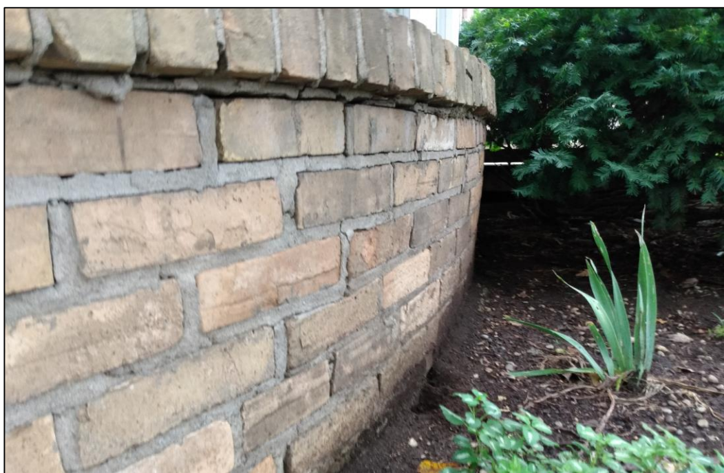
Figure 3: Close-up of mortar joint below bay window sill, showing mortar separating from brick and additional signs of animal burrowing. Source: City Staff.
