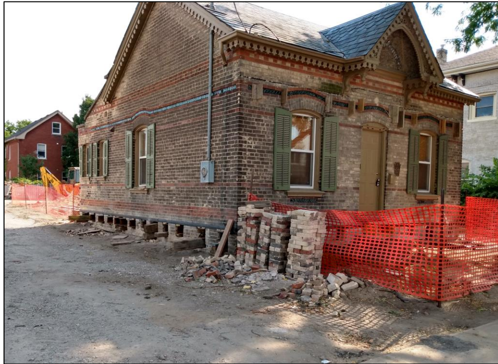
Figure 4: The front and east side of the Crystal Cottage showing the removal of the front porch as well as the installation of steel beams below the first floor, in preparation for the proposed relocation. Source: Staff.
