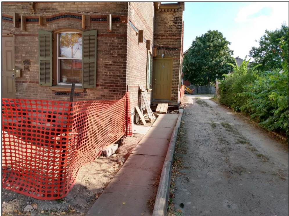
Figure 3: West side of the Crystal Cottage, showing that the front and side porches have been removed ahead of proposed relocation. Source: Staff.
