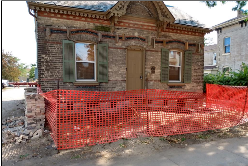
Figure 3: West side of the Crystal Cottage, showing that the front and side porches have been removed ahead of proposed relocation. Source: Staff.
