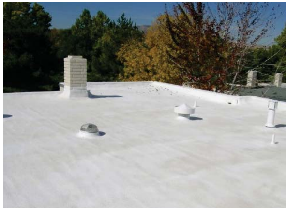
Light coloured roofs have a high solar reflectance, which reduces energy costs and the urban heat island effect.
