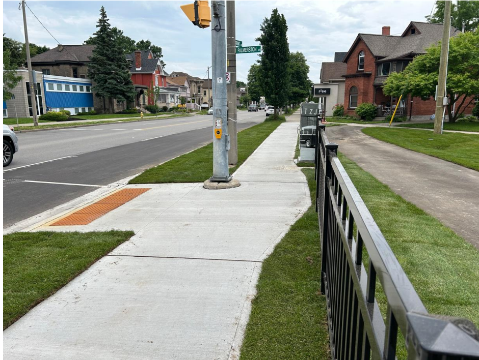
Figure 2 - Palmerston Street and Brant Avenue New Sidewalk and Tactile Walking Surface Indicators
