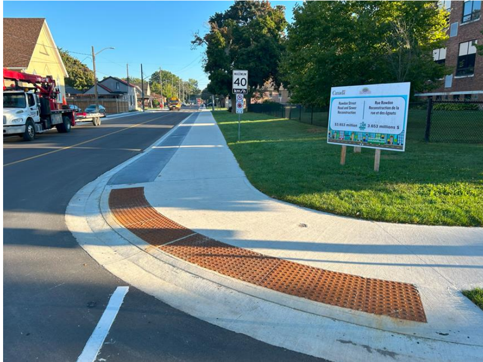
Figure 1 - Rawdon Street New Sidewalk and Tactile Walking Surface Indicators
