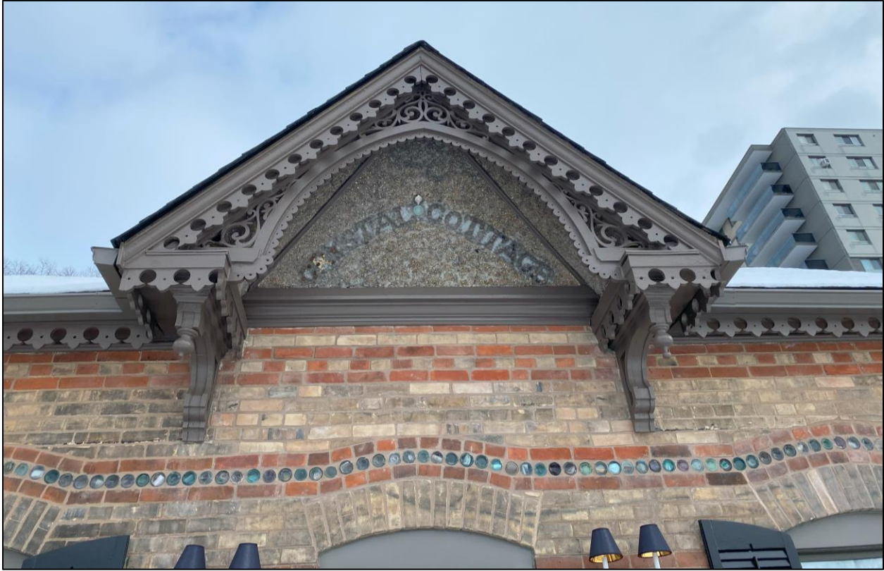
Figure 4: Close-up of the front gable showing the words "Crystal Cottage" as well as ornate wooden trim. On the brick wall below, part of the polychromatic brickwork is visible together with the course of glass bottles.
