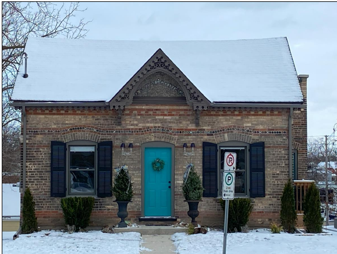
Figure 1: The restored Crystal Cottage at 53 Charlotte Street with the front façade as seen from Charlotte Street.
