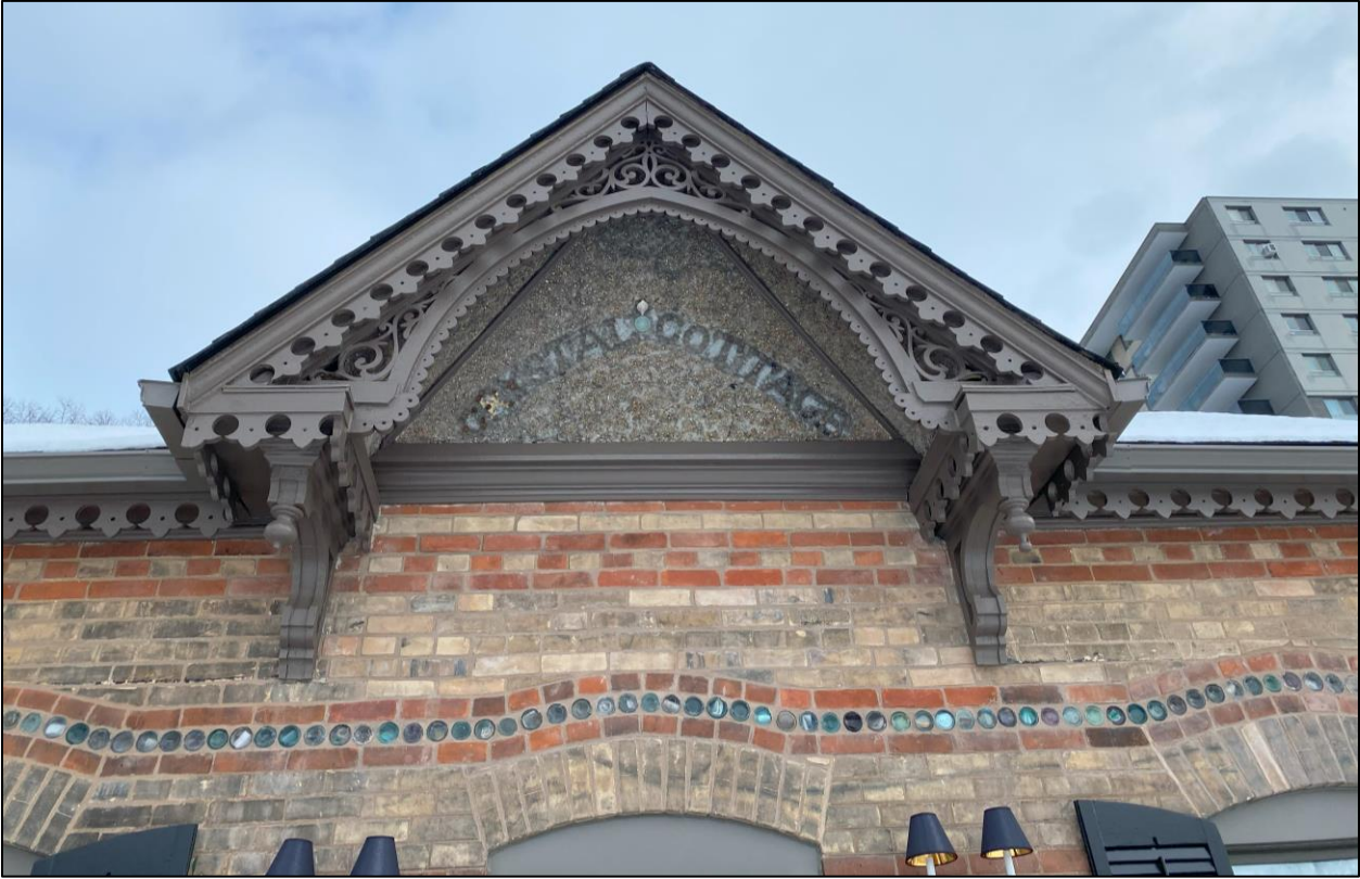
Figure 4: Close-up of the front gable showing the words "CRYSTAL COTTAGE" as well as ornate wooden trim. On the brick wall below, part of the polychromatic brickwork is visible together with the course of glass bottles.
