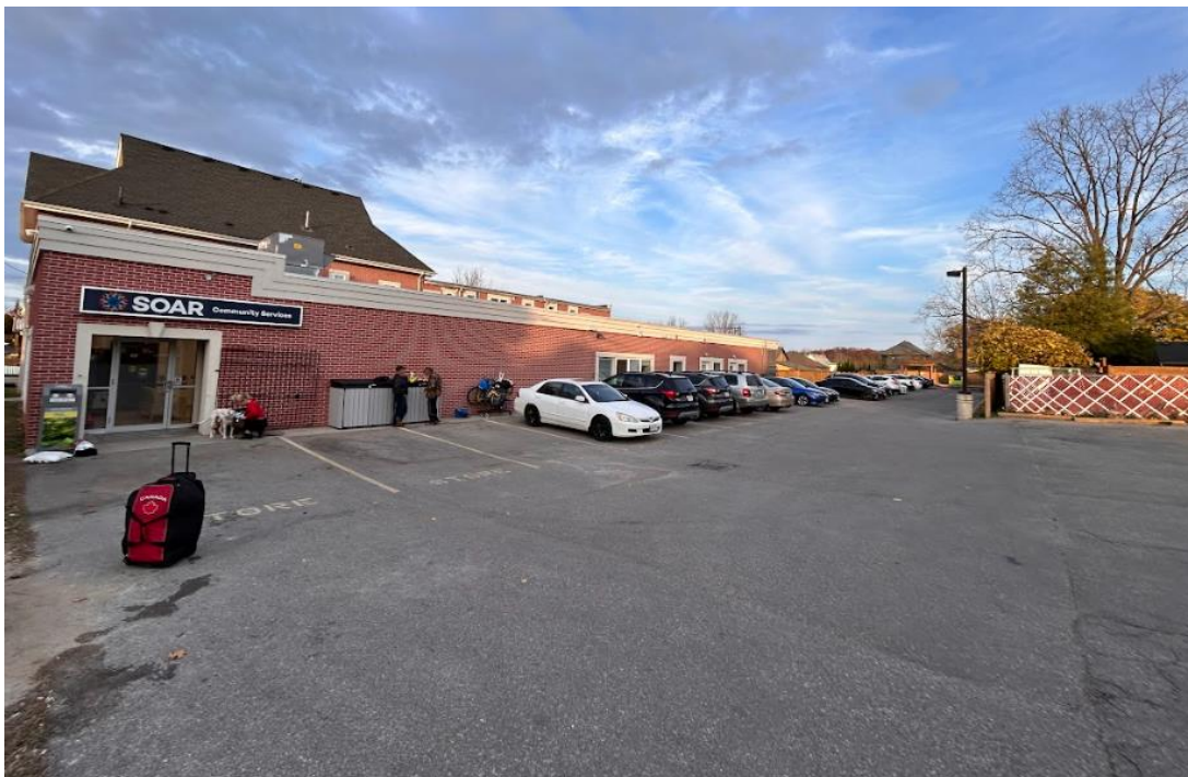
Figure 3 – Photo of Subject Lands – Resource Centre on 73 Murray Street
