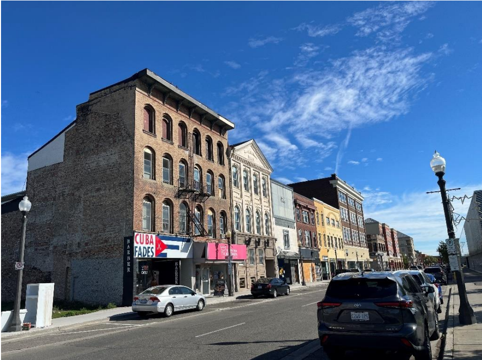
Plate 2: The north side of Colborne Street east of King Street (A.S.I., 2024).
