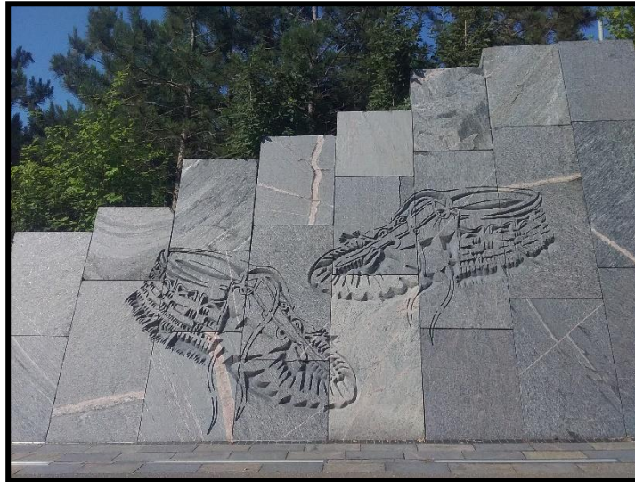
Plate 2: Moccasin Installation on Bridge in Trillium Park (ARA 2020)
