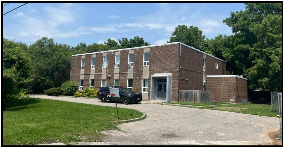
Figure 1 – Existing Apartment Building
