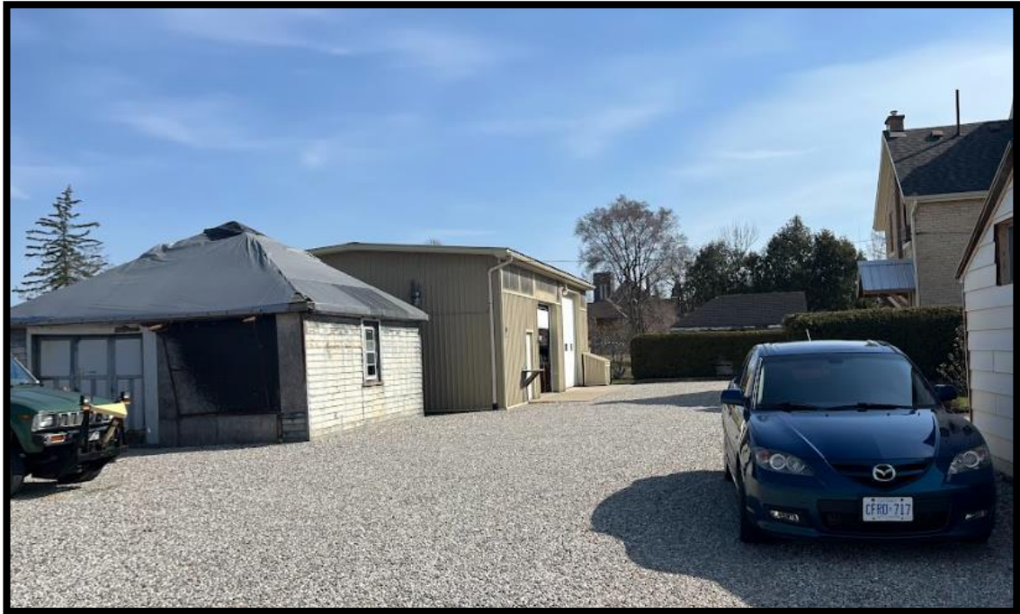
Figure 2 - Existing Accessory Buildings
