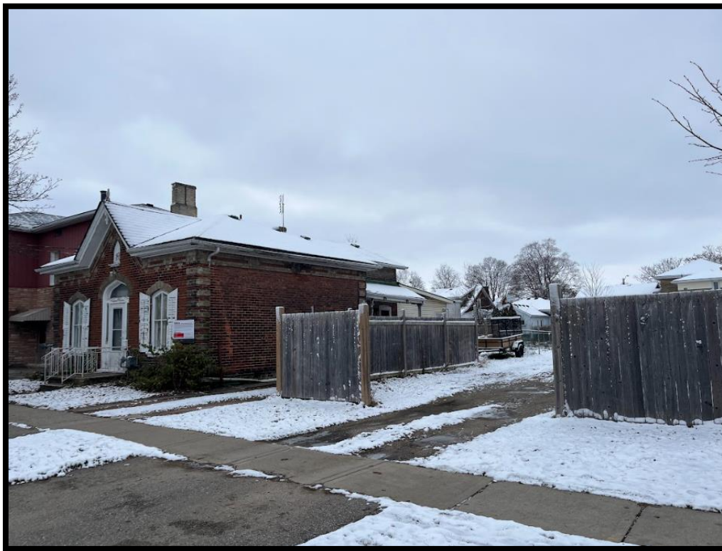
Figure 3 - Site visit view
