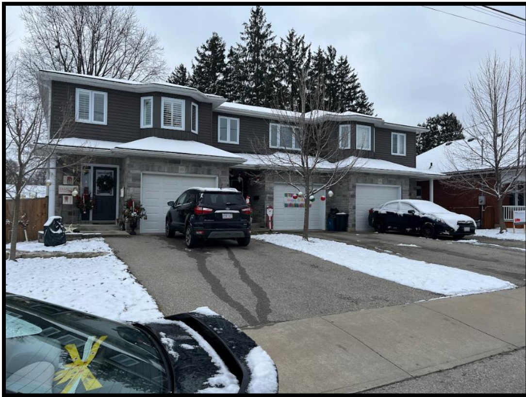
Figure 3 – Site visit view
