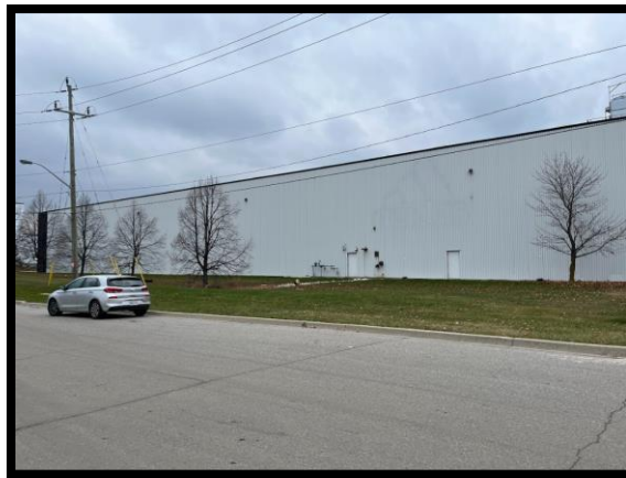
Figure 4 – View of the proposed battery location
