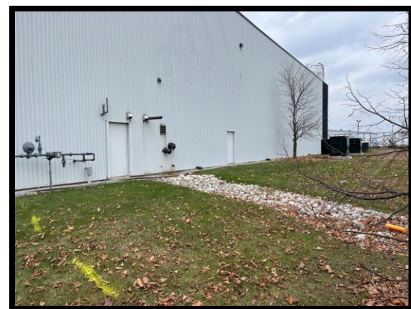
Figure 5 – View of the proposed battery location
