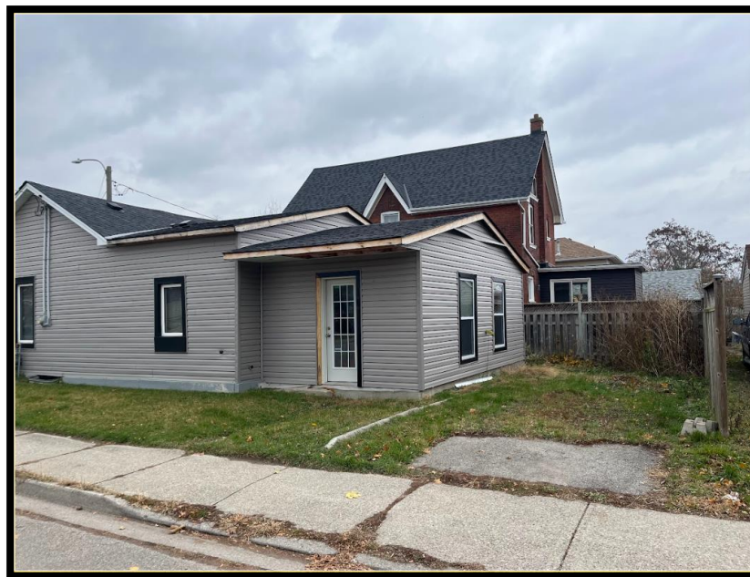
Figure 4 - View of the subject property
