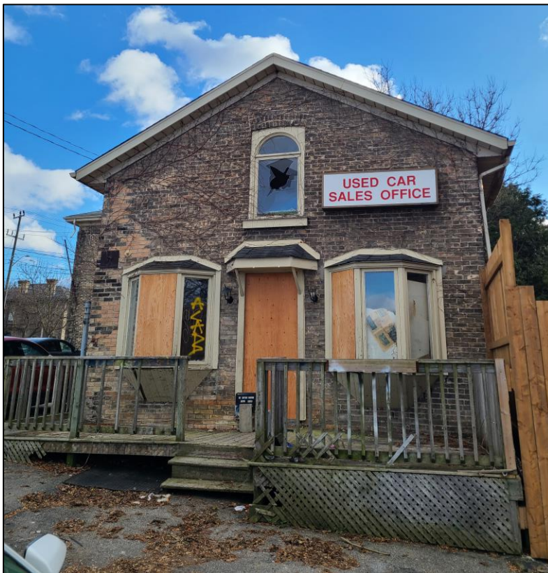
Figure 3 – Detached accessory structure located at 70 Alfred Street. Date: December 13, 2023.
