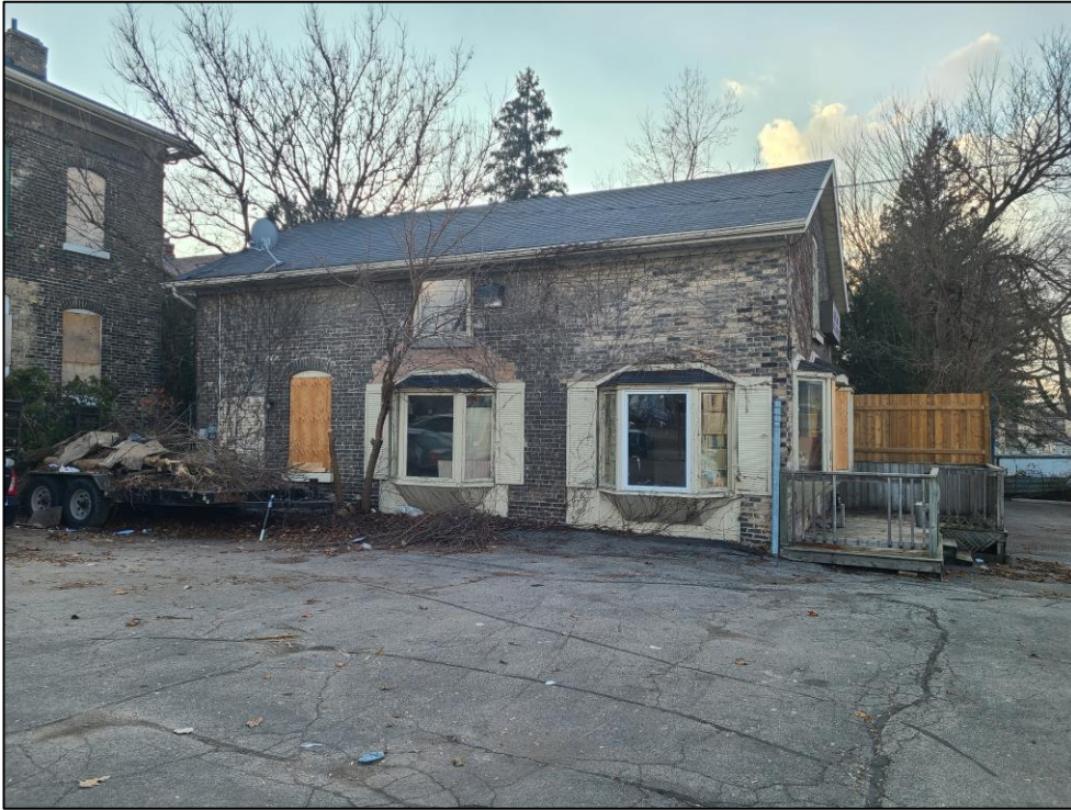
Figure 2: Detached accessory structure located at 70 Alfred Street. Date: December 13, 2023.
