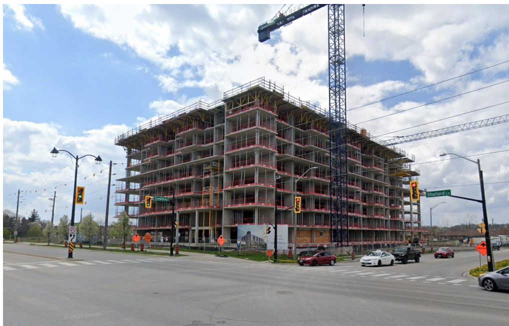
Figure 5 - View of the subject property under construction.
