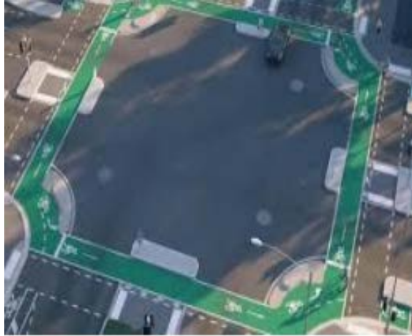
Figure 11: Image of a Protected Intersection
