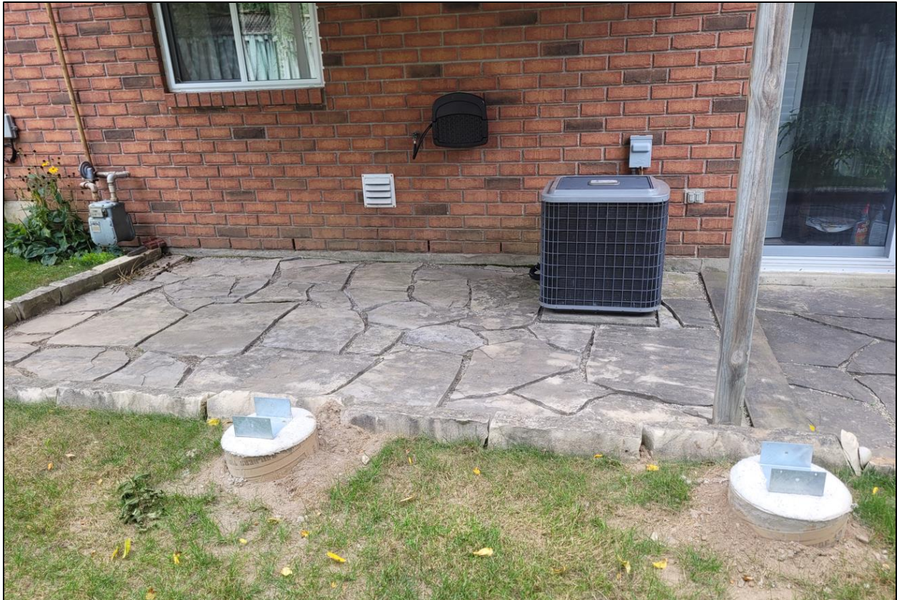
Figure 6 - Location of the new footings in relation to the existing footings and deck structure
