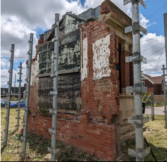
Photo 1: Cracking, deteriorated masonry and joints.
