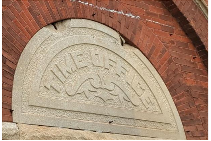
Photo 8: Deteriorated stone medallion and exposed dowels.
