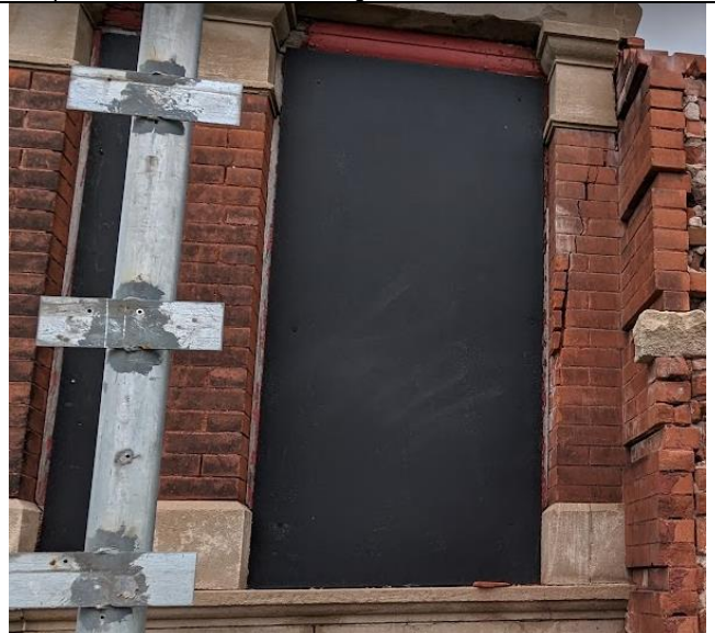
Photo 4: Boarded window and cracking brick
