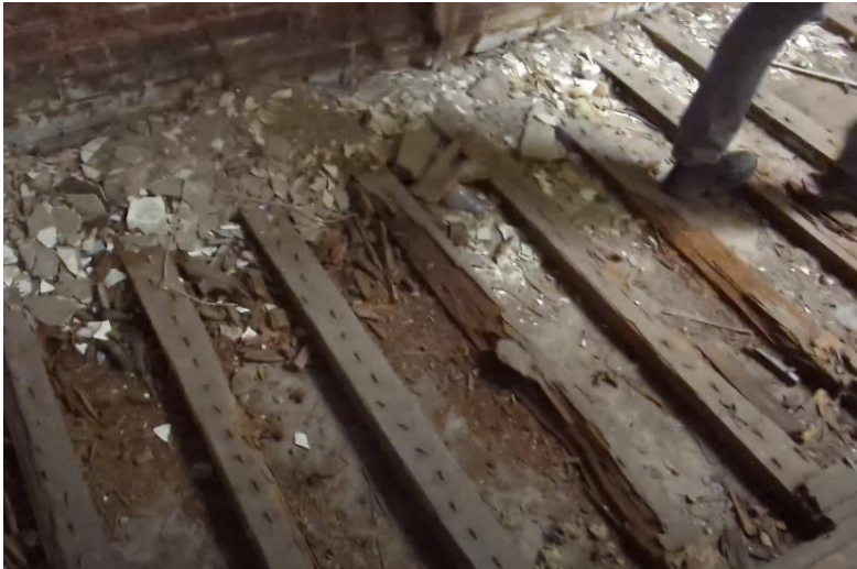
Photo 16: Deteriorated wood flooring.
