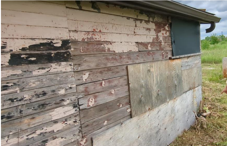
Photo 9: Deteriorated wood siding.
