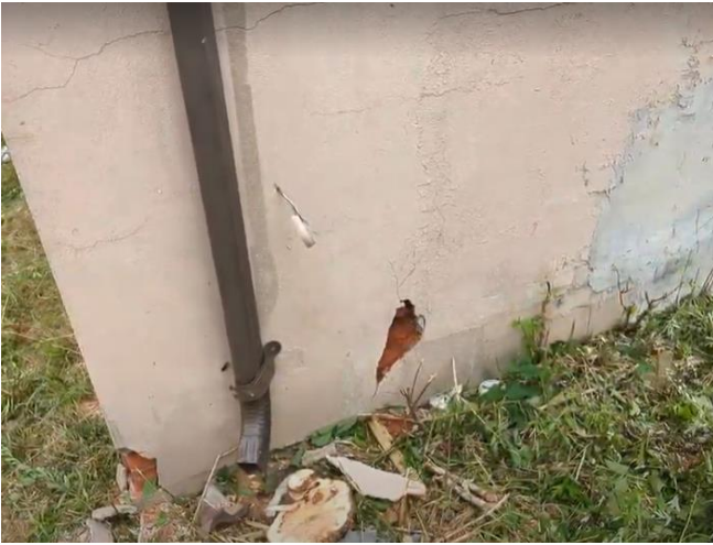
Photo 7: Delaminated parging and deteriorated brick behind.
