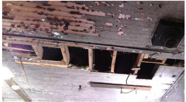
Photo 10: Exposed roof joists.
