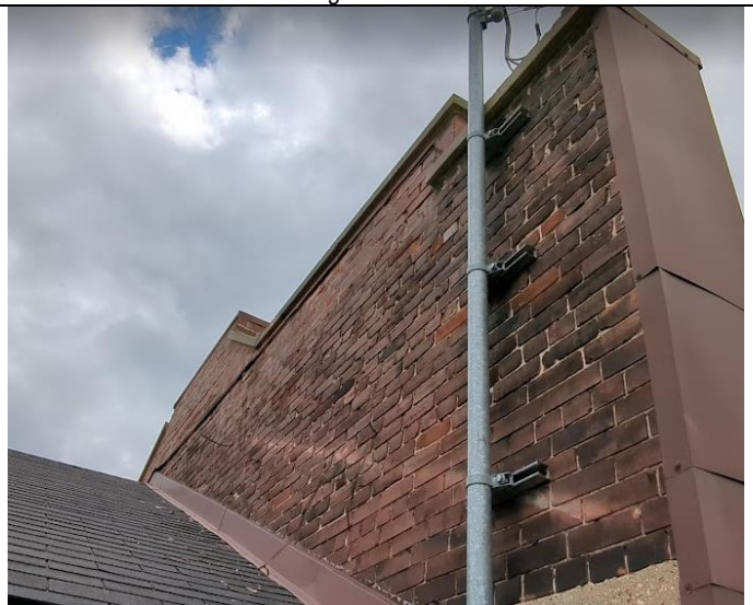
Photo 6: Cracking, deteriorated masonry and joints.
