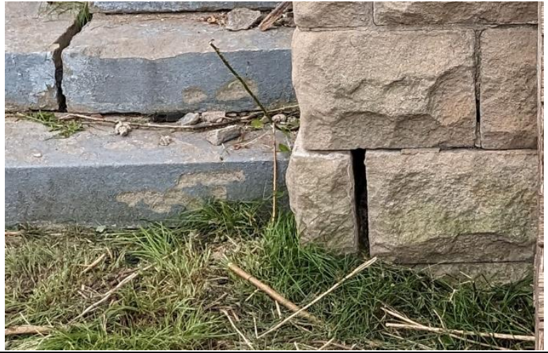
Photo 2: Displaced lower stone and missing mortar.
