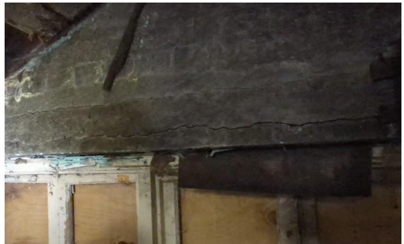
Photo 12: Deterioration of concrete lintel.
