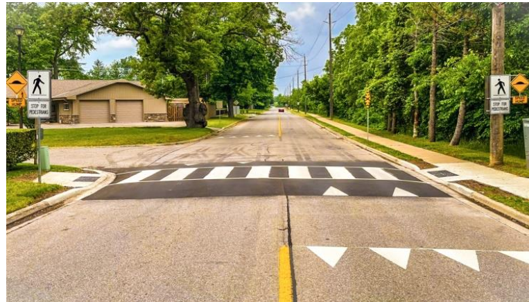
Raised PXO Crosswalk
