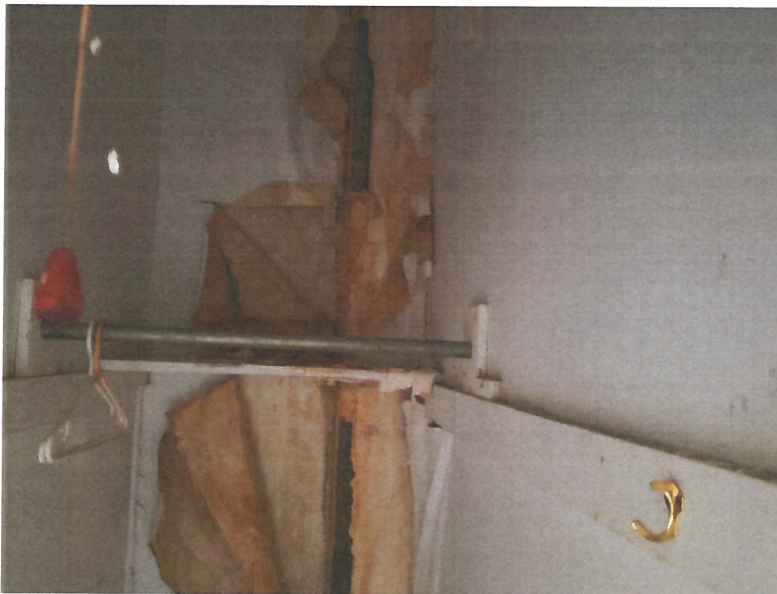
Photo No. 27 – Further evidence of water penetration in the upper levels of the residence.
