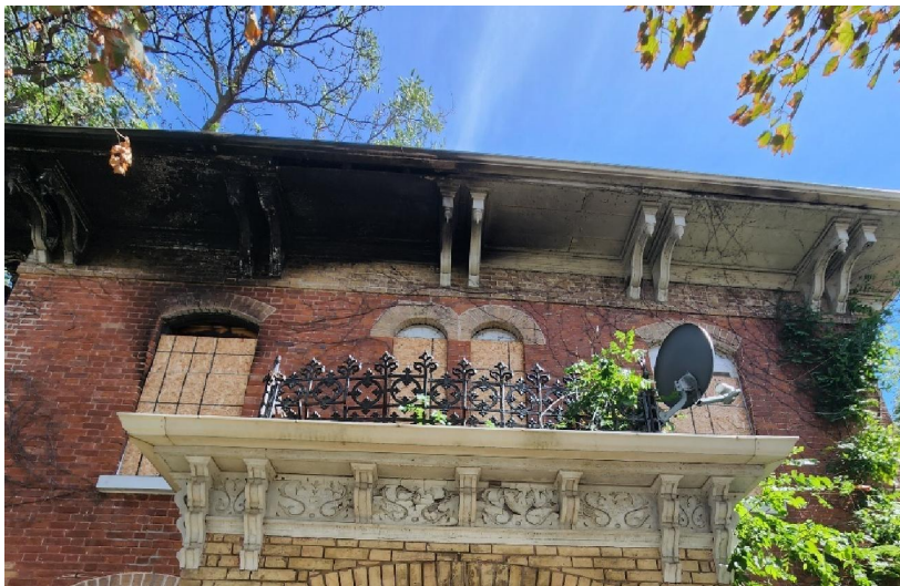
Figure 4: Fire Damage at 93 West Street (September 2, 2022)
