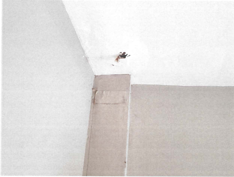
Photo No. 26 – Further evidence of water penetration in the upper levels of the residence.
