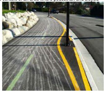
Figure 12: A hazard stripe painted around a lamppost in North Vancouver, BC.
