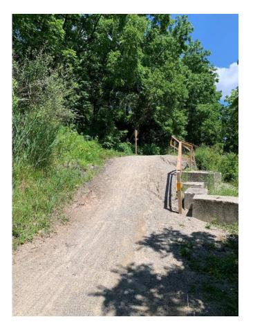
Figure 4. A steep limestone trail showing signs of erosion on the Hamilton-Brantford Rail Trail
