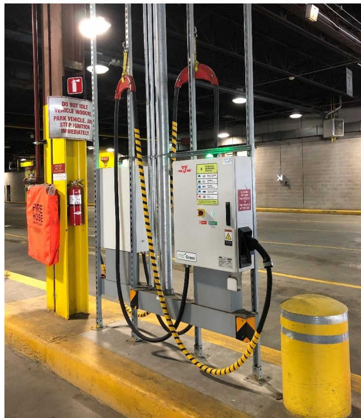
Exhibit 7: Example of two plug-in dispensers mounted on pad with drop-down conduits and protective bollard, serving charging spaces on both sides of the traffic island (Toronto Transit Commission)
