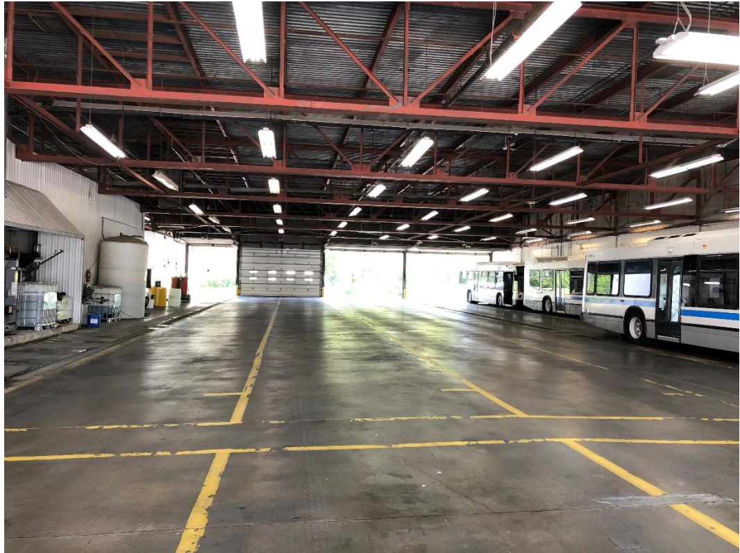
Exhibit 11: Lane 6 at Brantford Transit, showing walkway with minimal clearance
