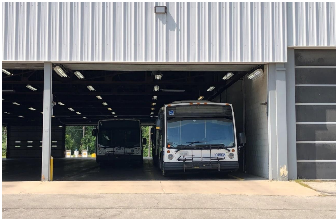
Exhibit 4: Exterior garage view showing double-width storage lane doorways and supporting columns
